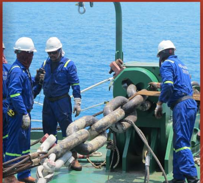
INSTALL CHAIN TO CHAIN STOPPER
