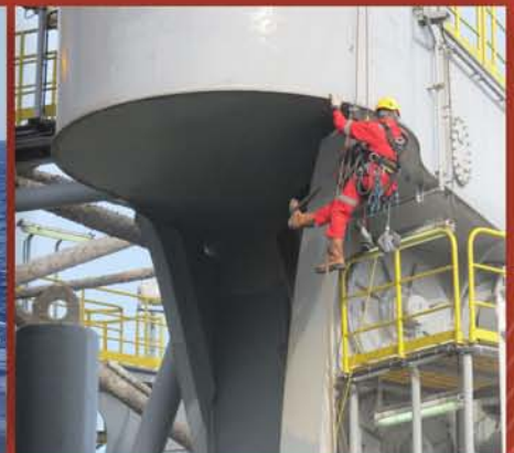
R.A.T. CONDUCT MPI INSPECTION RIG HYSY937 (Terminal Peti Kemas SBY, Th. 2021)
