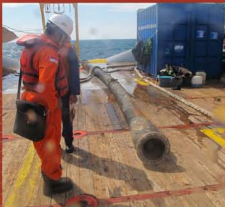
SUBSEA HOSE REPLACEMENT (PHEWMO, Poleng Field, Th. 2013)
