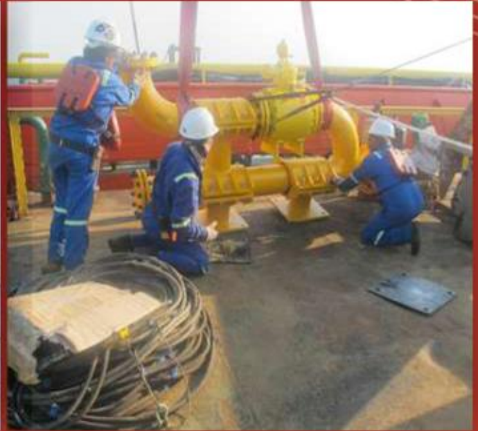
INSTALLATION OF SPOOL PIECE AT PLEM
