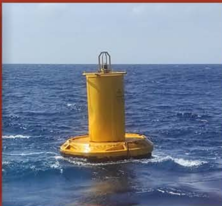
NAVIGATION BOUY INSTALLATION - SAKA INDONESIA PANGKAH LTD
