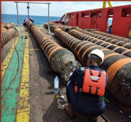
FLOATING HOSE INSTALLATION & REPLACEMENT (FSO KAS III, HCML Field, Th. 2020)
