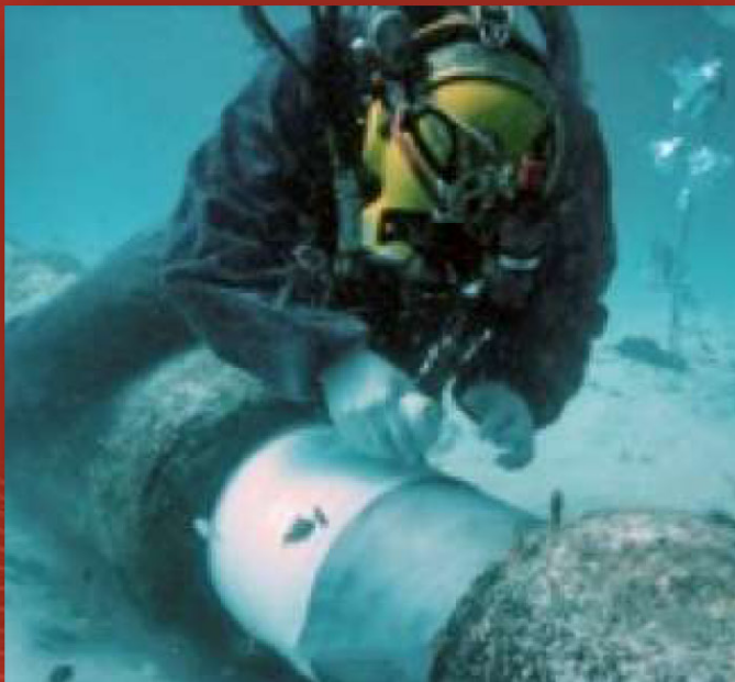
PIPELINE CONCRETE REMOVAL FOR NDT TEST
